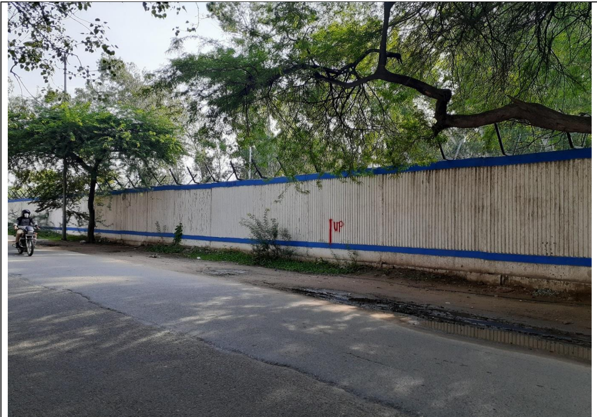
Photo 4 – Boundary wall of Tughlakabad Air Force Station which is located inside the Eco-Sensitive Zone. The line drawn in red on the boundary wall indicates the location of proposed underground tunnel.
