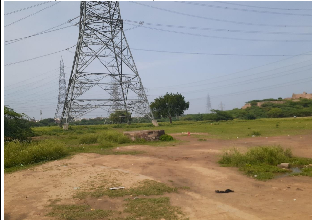
Photo 3 –Transmission tower located inside the Eco-Sensitive Zone. The proposed alignment passes beneath the open ground.
