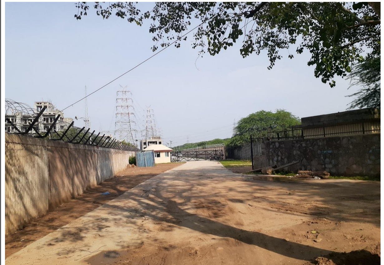
Photo 5 – Gate of Sub Station which is located inside the Eco-Sensitive Zone.
