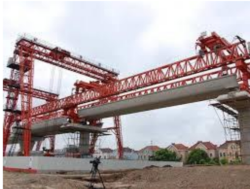
Figure 2: Placing full precast span (with launching girder)
