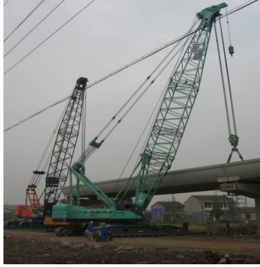
Figure 1: Placing full precast span (with crane)
